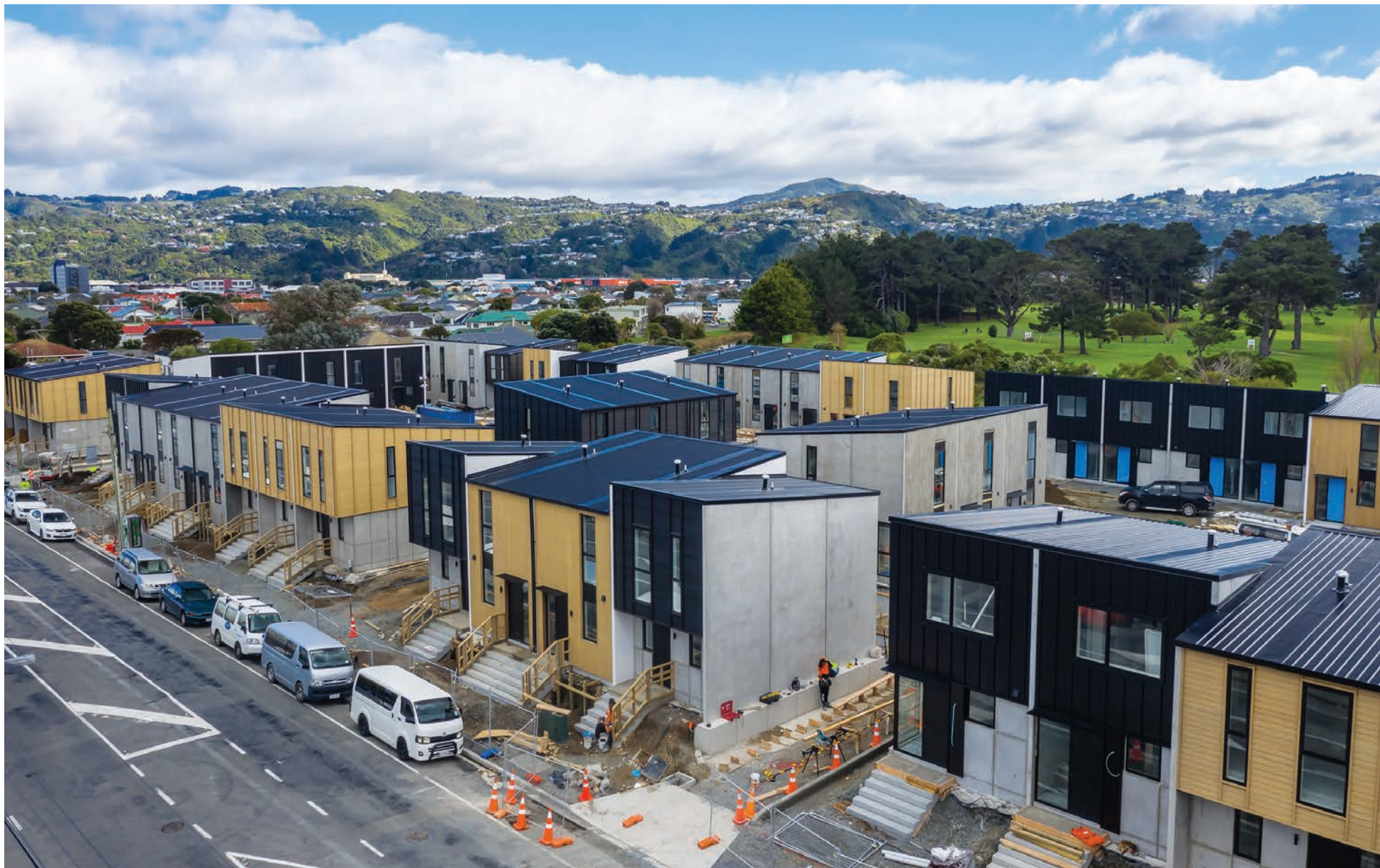
Paetutu development in Petone includes 56 terraced two-level homes constructed with Homestead's precast construction method.
